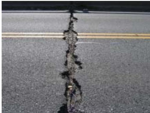
Bridge joint movement exceeds the asphalt’s ability to expand and contract. With the joint opened up, water, salt and chemicals can corrode steel girders and bearings underneath. This movement also causes the asphalt to break apart putting debris on the bridge deck. Not only is this a windshield hazard, but it can create a pot hole like effect across the entire bridge.
