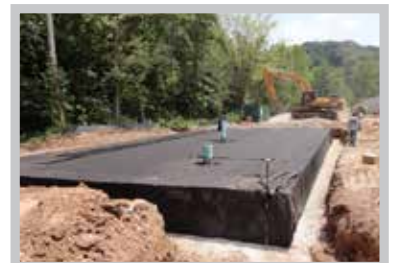
Fig. 21 Finished envelope should lay flat against R-Tank®.
