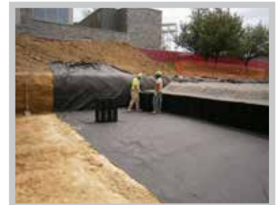
Fig. 5 Pull wrinkles out of geotextiles so material lays flat.
