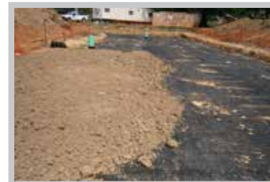
Fig. 26 Pushing backfill parallel to the Geogrid prevents the grid from shoving.
