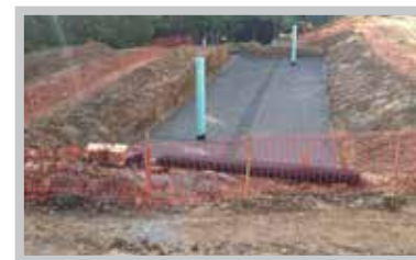
Fig. 27 Secure the installation with temporary fencing.
