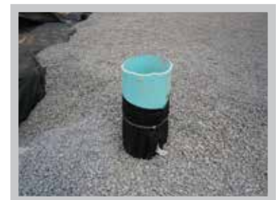
Fig. 17 Install port into R-Tank®.
