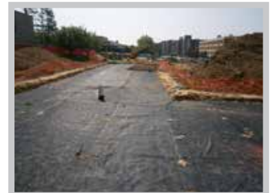
Fig. 25 Overlap Geogrid 18" or as required by plans.
