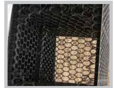
Fig. 15 If after adjusting the internal plates, the pipe will not fit, the top plate can be cut off-center and one of the internal plates can be removed.
