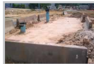
Fig. 28 Secured R-Tank® installation using Jersey Barriers.
