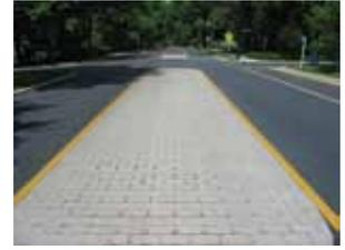
Patterned Pavement products are a hot applied synthetic asphalt material that bonds permanently to the surface. If you want the look of brick paving, but want it to last many years without any maintenance, then Patterned Pavement is the solution.
